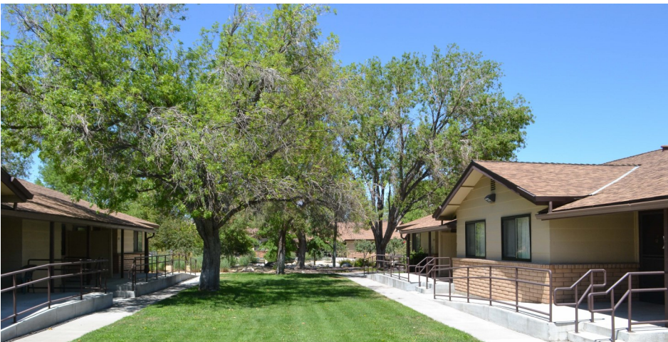
Like the Silverada Complex, the RHA ensures all housing units are well maintained and are safe communities.
