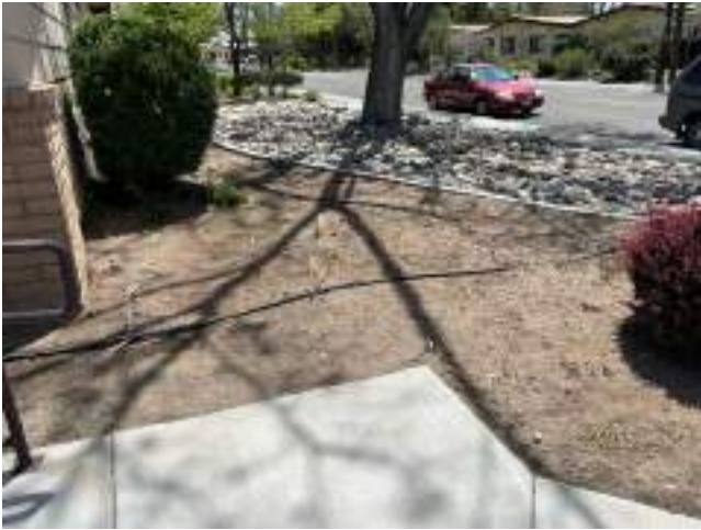
29. Barren Landscaping Near Building 16 (Non-Critical Repair)
