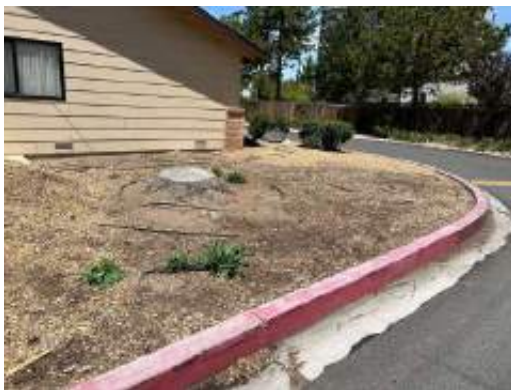
Barren Landscaping Near Building 7 (Non-Critical Repair)
