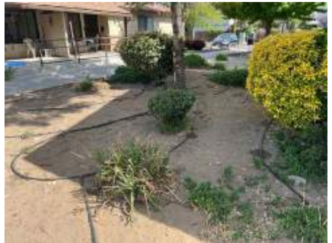
28. Barren Landscaping Near Building 1 (Non-Critical Repair)
