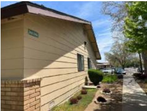
Exterior Wood Siding
