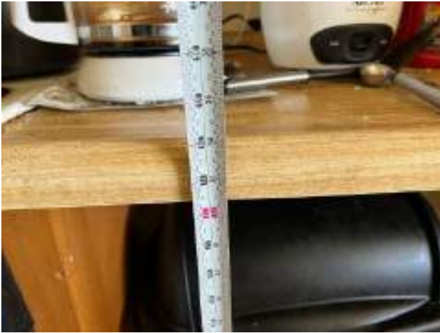
5. HDCP Unit 2493 Bld 15 Studio - Kitchen Counter Height
