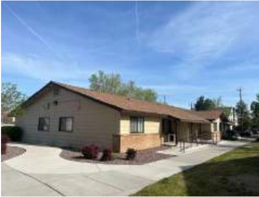
Typical Building Roof
