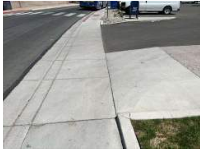
2. Concrete Entrance Apron
