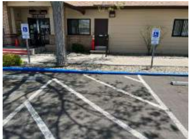
132. Construct Curb Cut to Sidewalk (Repair)
