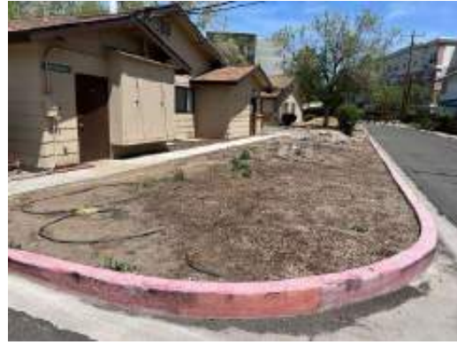
Barren Landscaping Near Building 7 (Non-Critical Repair)
