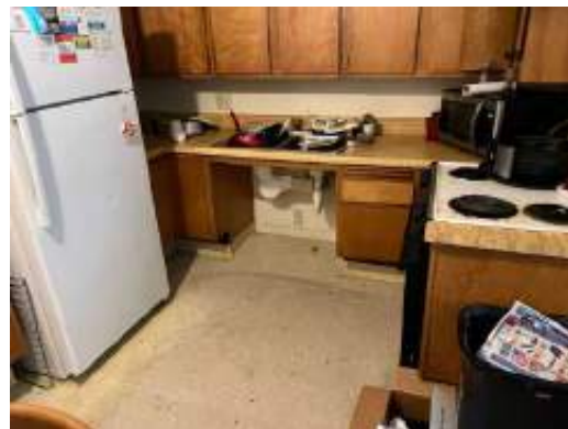
HDCP Unit 2601 Bld 9 2 Bed 1 Bath - Kitchen (Repair)
