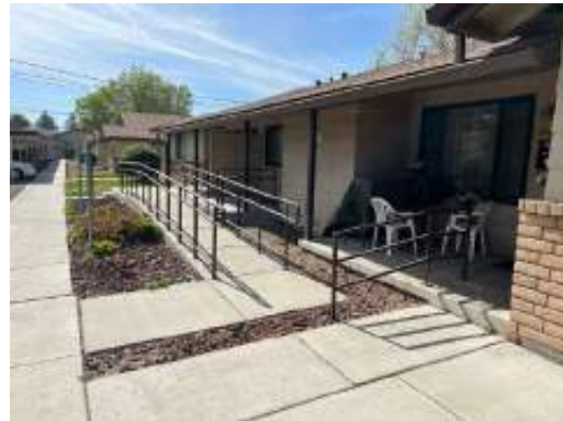
Ramp at Unit Entry
