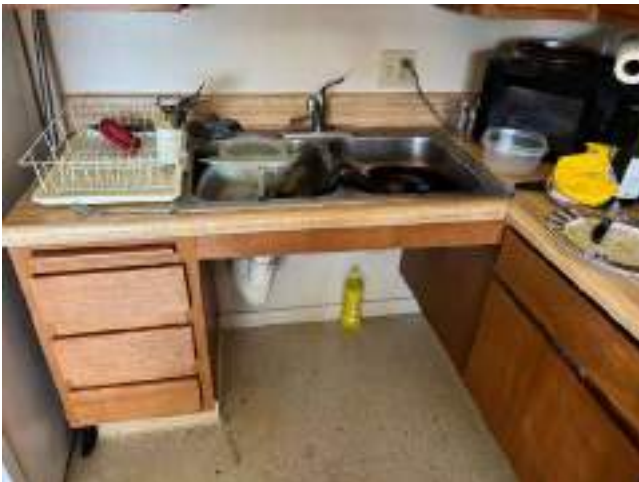
7. HDCP Unit 2493 Bld 15 Studio - Kitchen Sink
