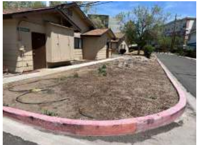
32. Barren Landscaping Near Building 7 (Non-Critical Repair)
