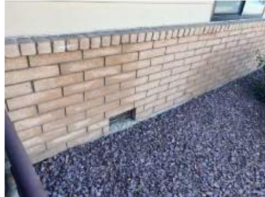
Crawl Space Vent
