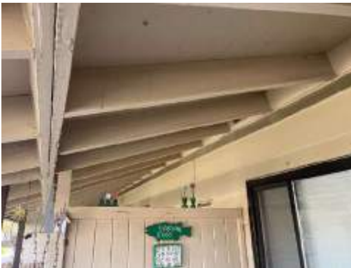
Roof Overhang at Unit Patios
