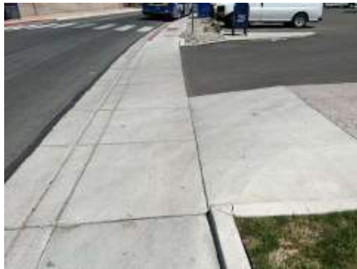
Concrete Entrance Apron
