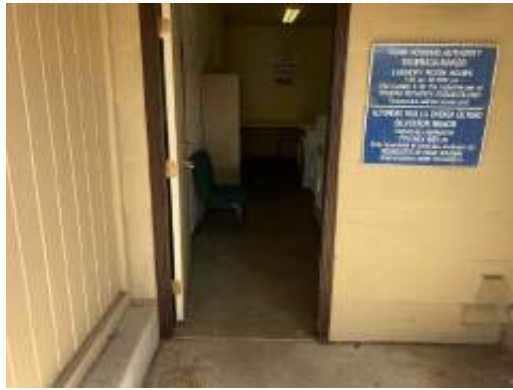
Laundry Room Entry
