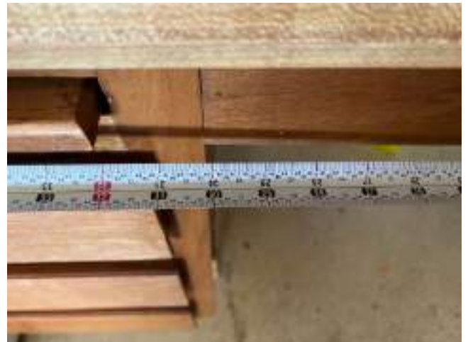
8. HDCP Unit 2493 Bld 15 Studio - Sink Width
