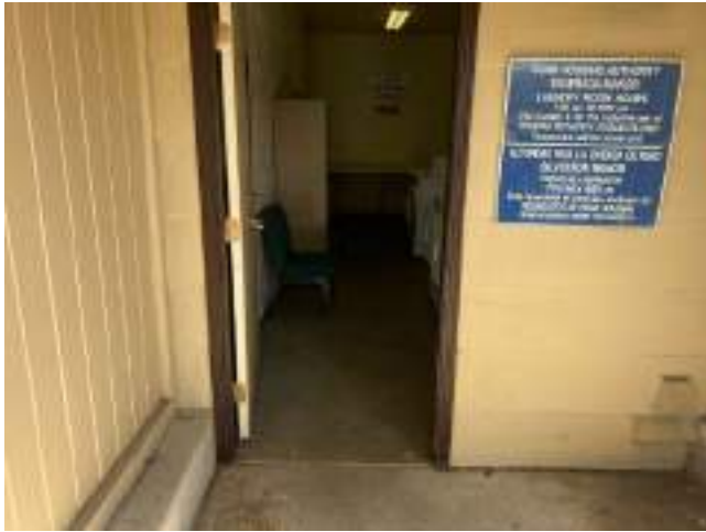
105. Laundry Room Entry
