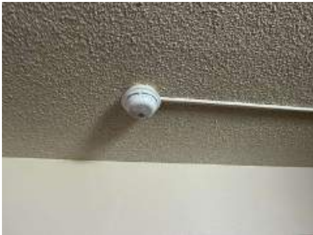
91. Hard Wired Smoke Detector
