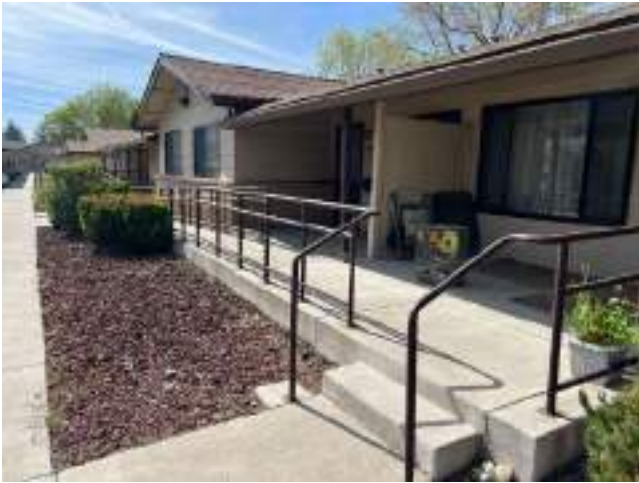
13. Concrete Ramp and Stairs at Apartment Entry
