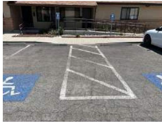
Access Aisle at ADA Stalls
