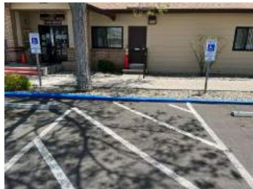
Construct Curb Cut to Sidewalk (Repair)
