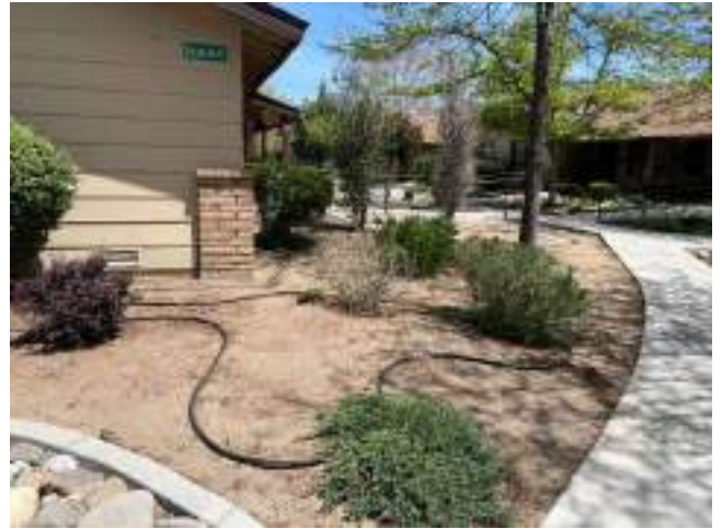
30. Barren Landscaping Near Building 16 (Non-Critical Repair)
