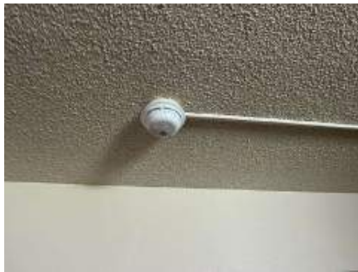
Hard Wired Smoke Detector
