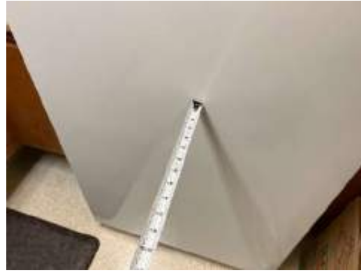
HDCP Unit 1438 Bld 2 2 Bed 1 Bath - Counter to Fridge (Repair)
