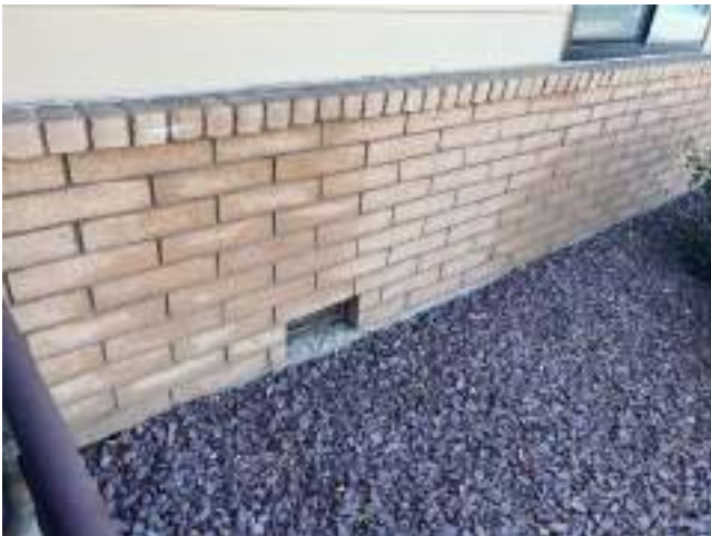
51. Crawl Space Vent
