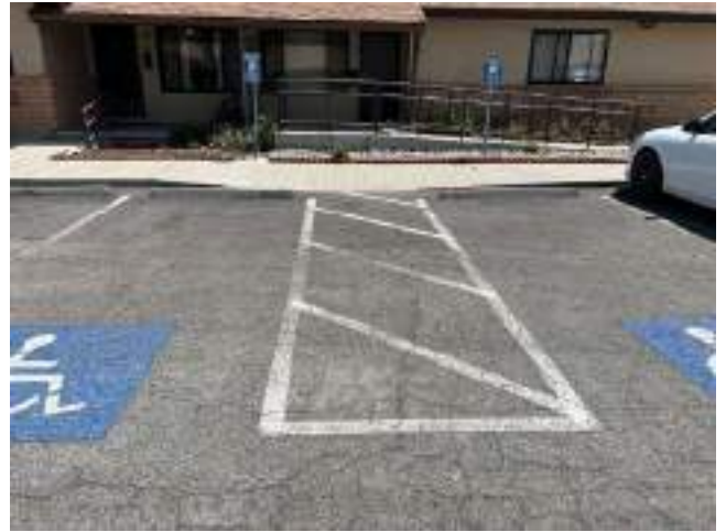
130. Access Aisle at ADA Stalls
