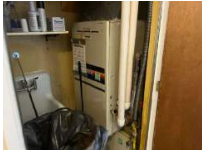
84. Common Area Fan Coil Unit
