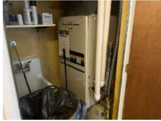
Common Area Fan Coil Unit
