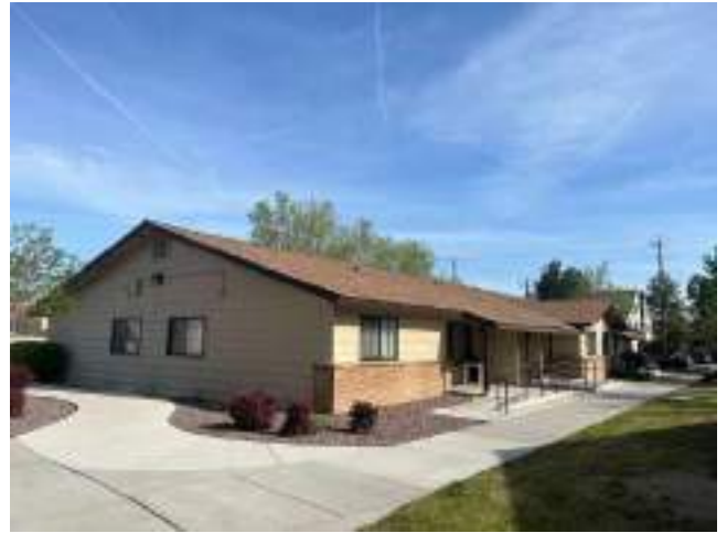
66. Typical Building Roof
