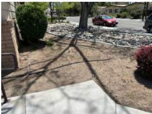
Barren Landscaping Near Building 16 (Non-Critical Repair)
