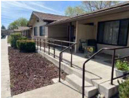
Concrete Ramp and Stairs at Apartment Entry
