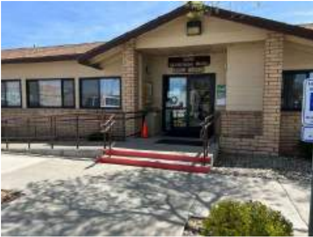
133. Entry Stairs at Community Center - Office
