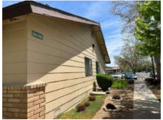
62. Exterior Wood Siding
