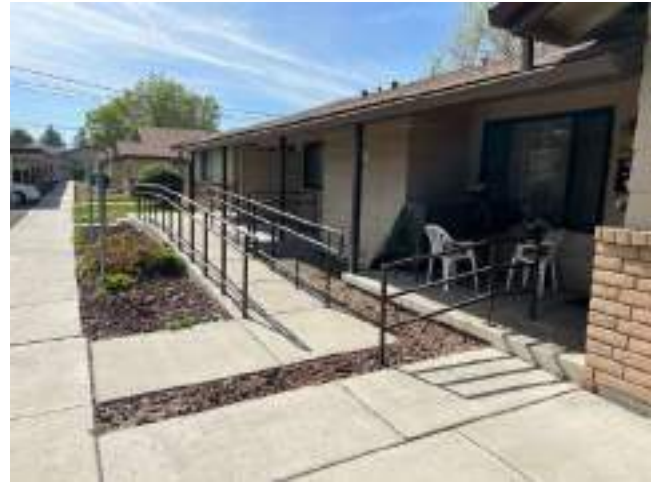
14. Ramp at Unit Entry
