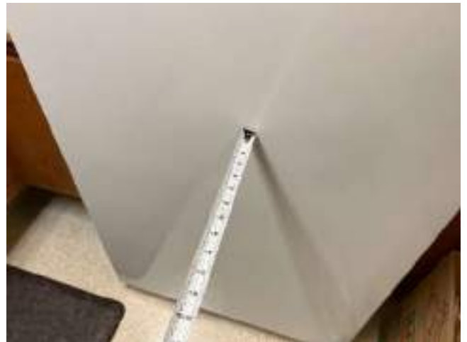
32. HDCP Unit 1438 Bld 2 2 Bed 1 Bath - Counter to Fridge (Repair)
