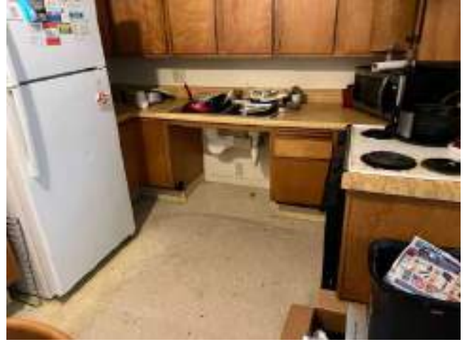
50. HDCP Unit 2601 Bld 9 2 Bed 1 Bath - Kitchen (Repair)
