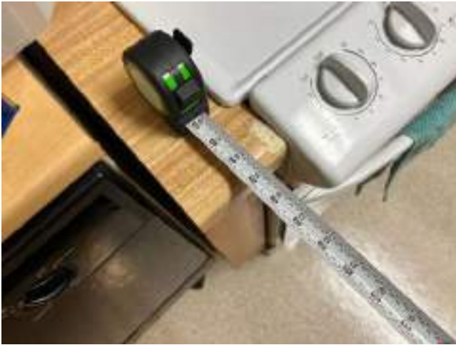
33. HDCP Unit 1438 Bld 2 2 Bed 1 Bath - Counter to Fridge (Repair)
