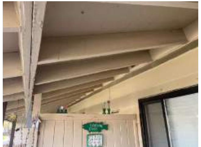
68. Roof Overhang at Unit Patios
