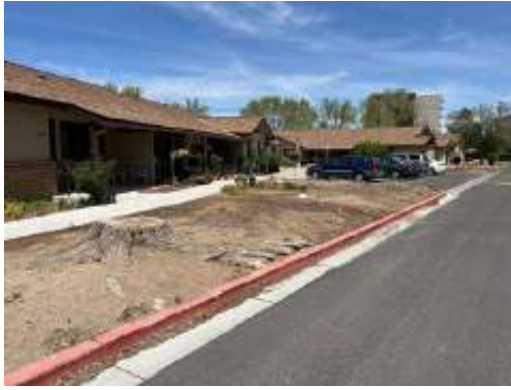
Barren Landscaping Near Building 8 (Non-Critical Repair)
