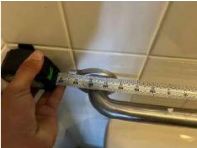
27. HDCP Unit 2605 Bld 9 1 Bed 1 Bath - Rear Grab Bar Width
