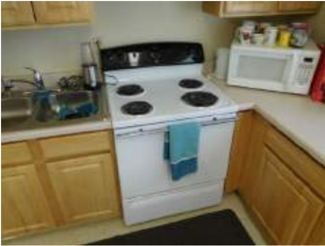
37. Leasing Office Community Room Kitchen non accessible kitchen range
