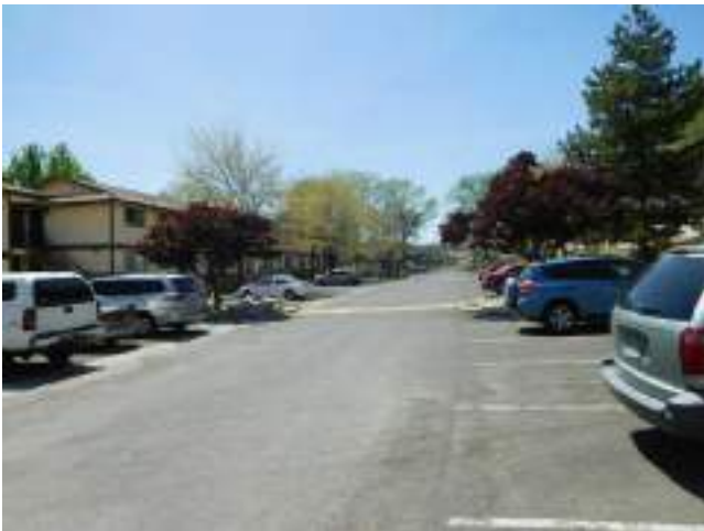
71. Typical asphalt paving
