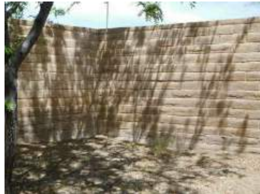
Partially retaining site wall at northern end of site
