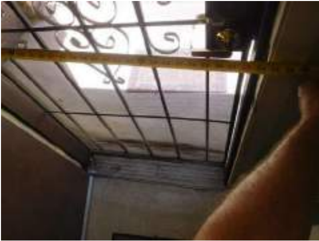
17. Bld 2541-Unit 1-2x1-UFAS -Entry at main door
