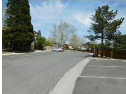
Typical asphalt paving
