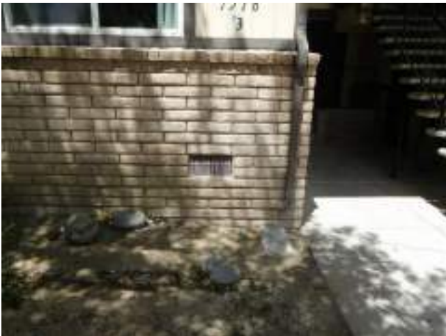
139. Representative crawl space venting
