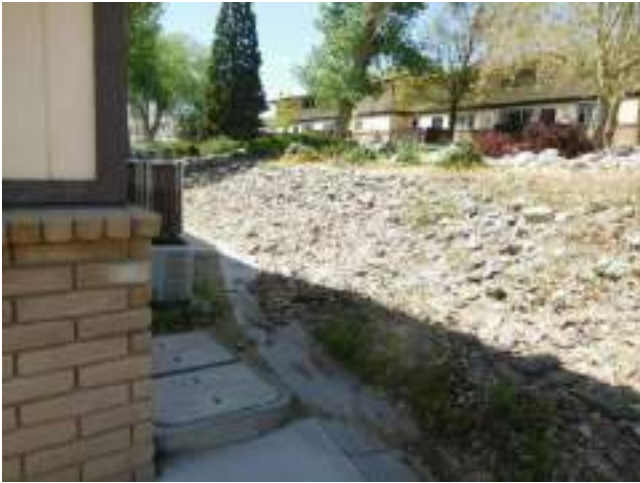
117. Wrip-wrap covered site slope
