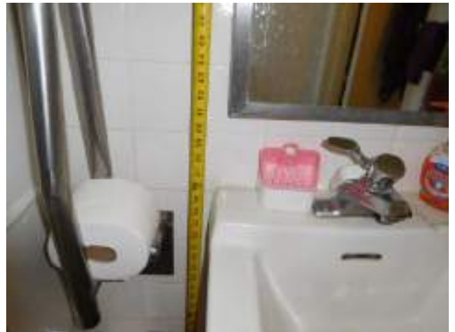
24. Bld 2541-Unit 1-2x1-UFAS -Bathroom
