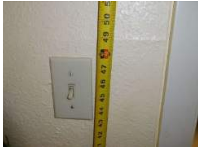
52. Leasing Office Community Room bathroom light switch
