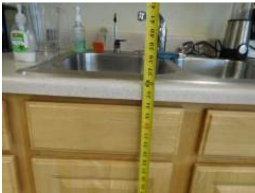
Leasing Office Community Room Kitchen non accessible kitchen sink
