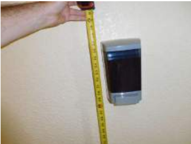
47. Leasing Office Community Room bathroom
