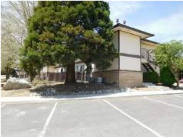
17. Typical exterior area
