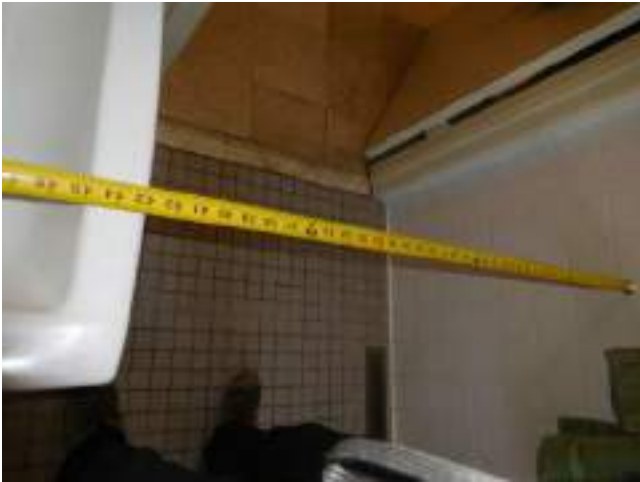
32. Bld 2541-Unit 1-2x1-UFAS -Bathroom
