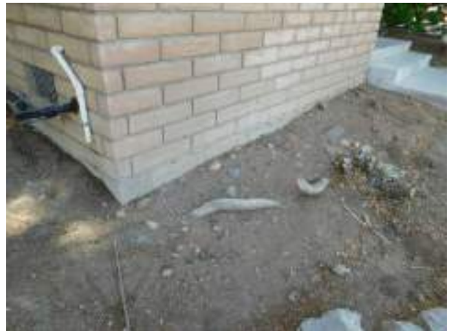
140. Masonry veneer CMU footing
