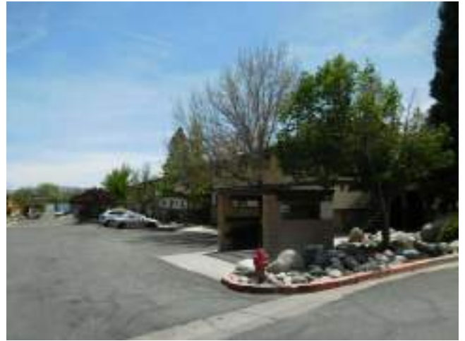
14. Typical exterior area
