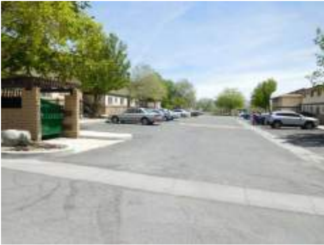
73. Typical asphalt paving
