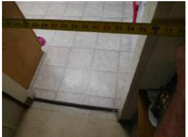
44. Bld 2541-Unit 1-2x1-UFAS -Kitchen entrance
