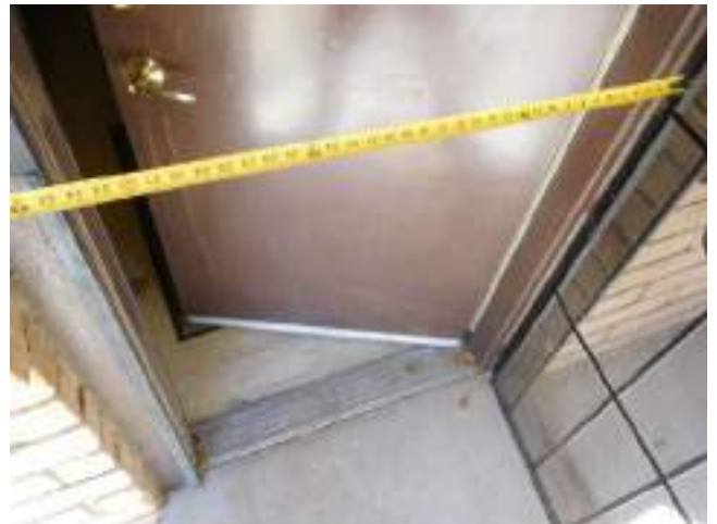
16. Bld 2541-Unit 1-2x1-UFAS -Entry at storm door
