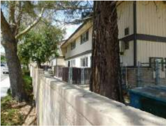
113. Site wall at southern end of site
