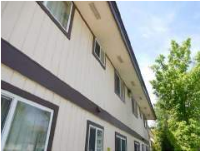
145. Facade with soffit venting
