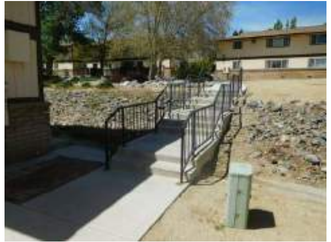
102. Site stairway north of 2539 and 2545 Buildings
