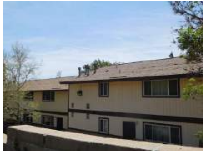
156. Typical roof condition
