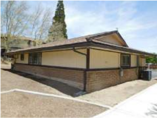
21. Leasing Office rear
