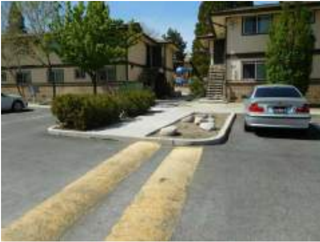
81. Typical flatwork termination at drive intersection
