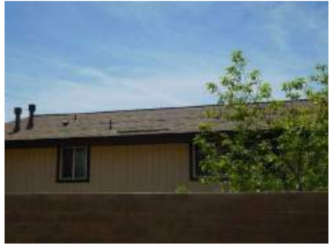
154. Typical roof condition
