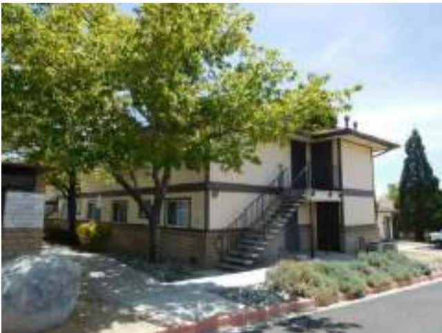
11. Typical exterior area
