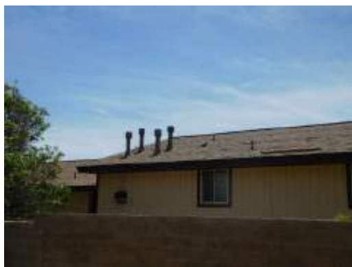
Typical roof condition
