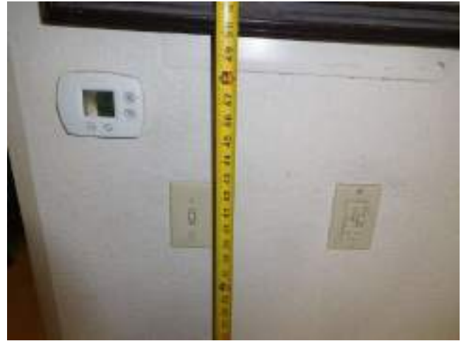
18. Bld 2541-Unit 1-2x1-UFAS -Typical wall switch and thermostat height
