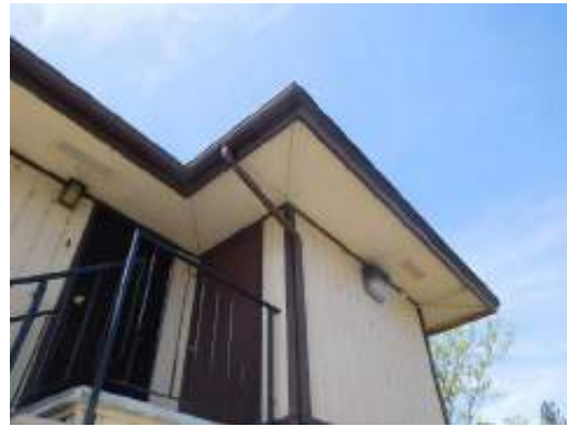
Facade with soffit venting
