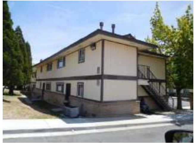
10. Typical exterior area
