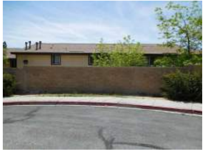
106. Partially retaining site wall at northern end of site
