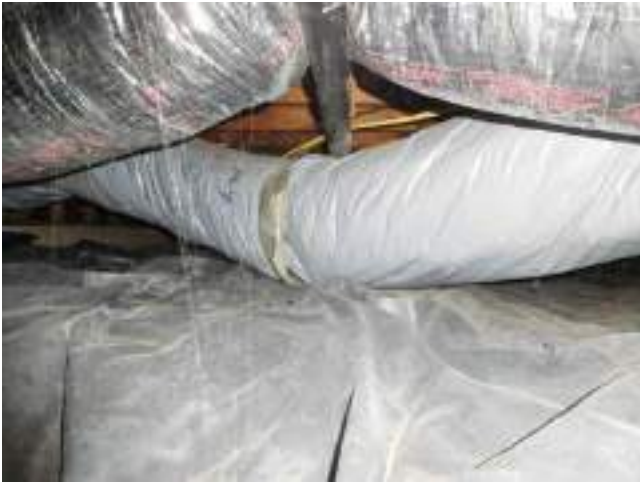
137. Representative crawl space with wood floor joists and moisture barrier
