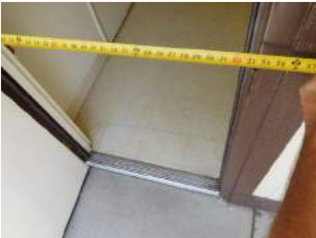
27. Leasing Office main entrance
