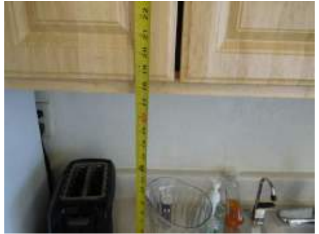
38. Leasing Office Community Room Kitchen upper cabinets
