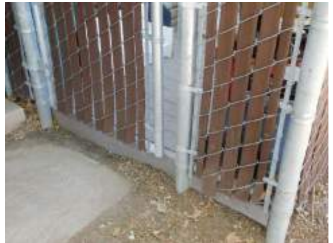
124. Ground level rear deck enclosed with chain linked fencing
