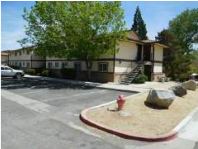
19. Typical exterior area
