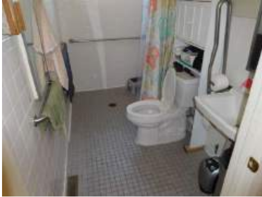
Bld 2541-Unit 1-2x1-UFAS -Bathroom
