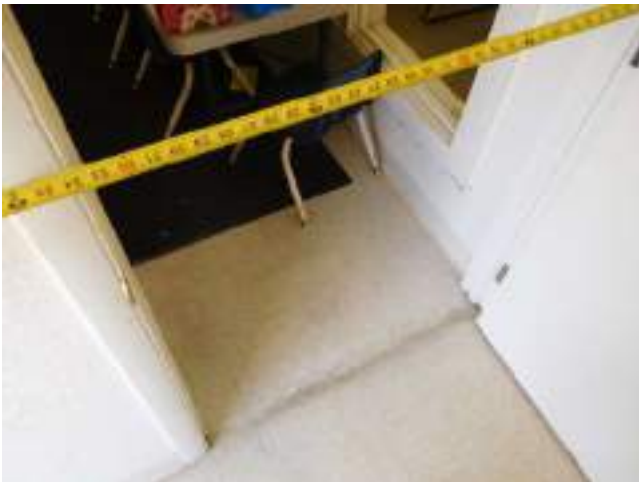
39. Leasing Office Community Room office entrance
