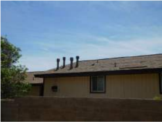
153. Typical roof condition
