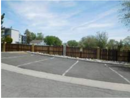
Typical asphalt paving
