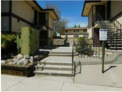
Site stairway between 2539 and 2545 Buildings
