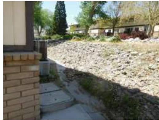
Wrip-wrap covered site slope
