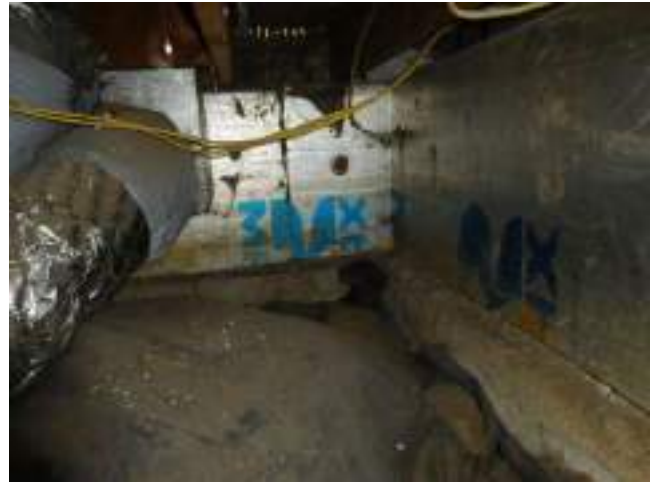
138. Representative crawl space
