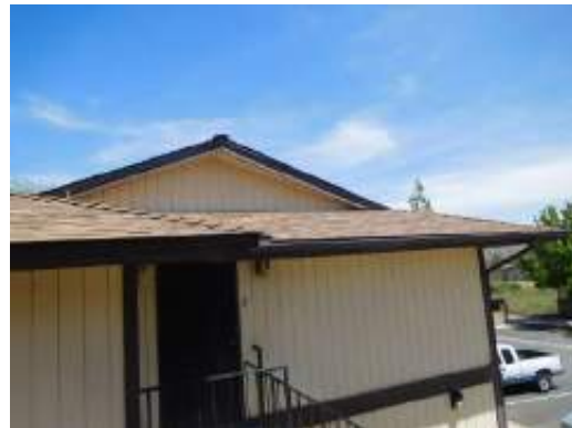
Typical roof condition with flashing
