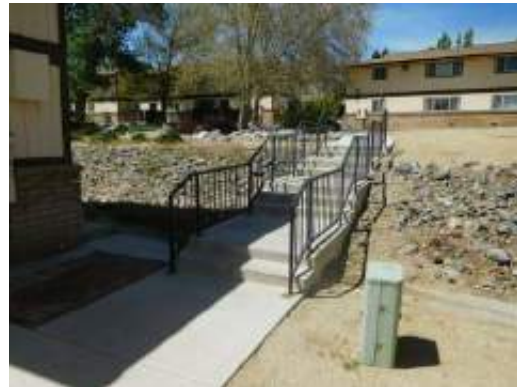
Site stairway north of 2539 and 2545 Buildings
