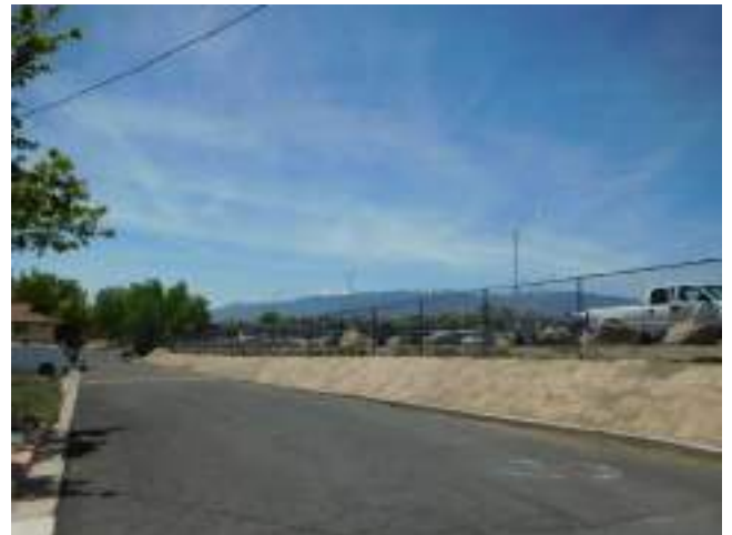
8. Western side of site northern end
