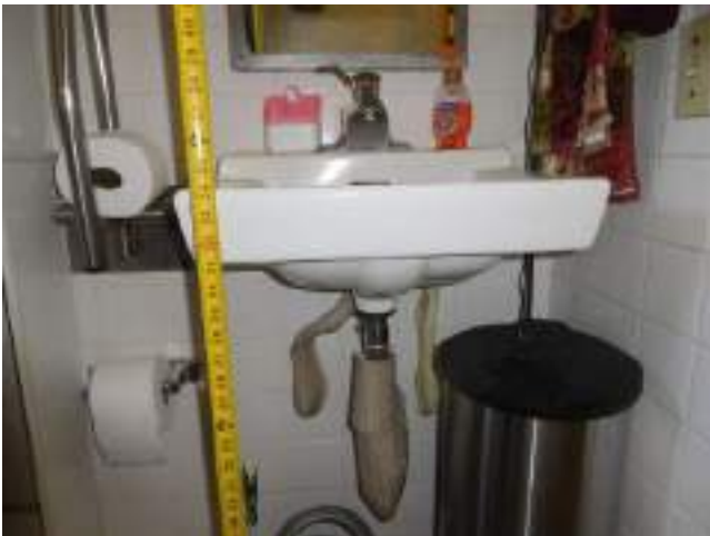
23. Bld 2541-Unit 1-2x1-UFAS -Bathroom
