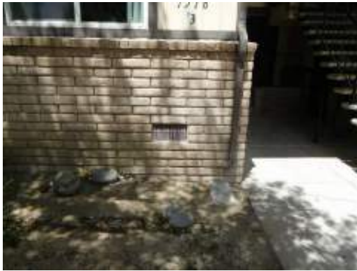
Representative crawl space venting
