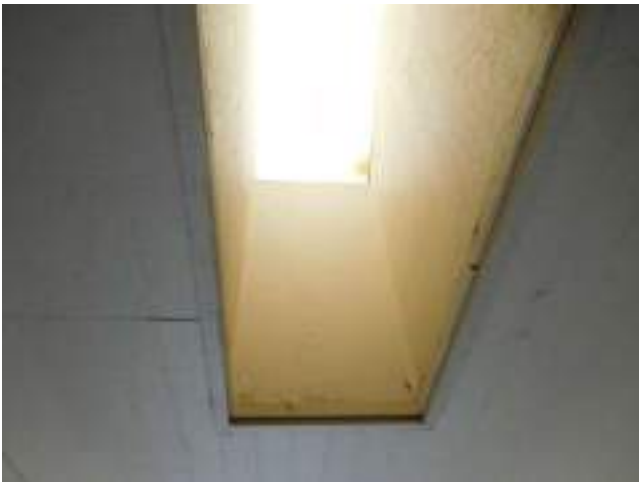
159. Typical roof skylight
