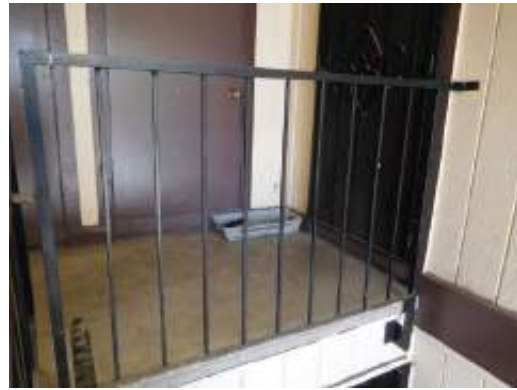
Typical onsite railing system
