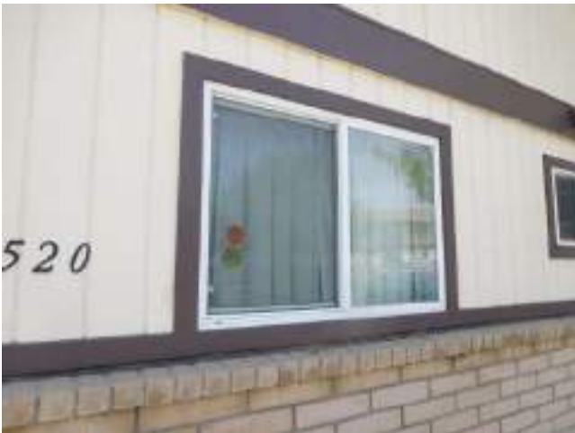
151. Typical window unit
