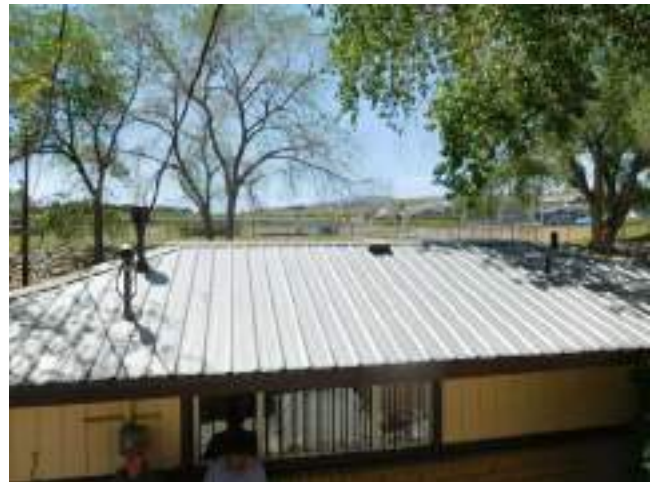
88. Laundry room metal panel roofing
