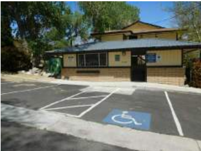
87. Laundry room with non-compliant access pathway from accessible space (Critical Repair)
