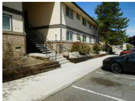
Landscaping timber retaining wall
