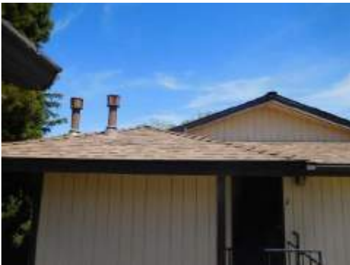
Typical roof condition
