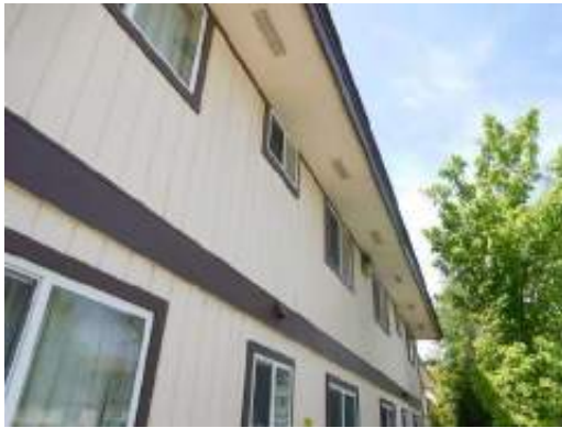
Facade with soffit venting
