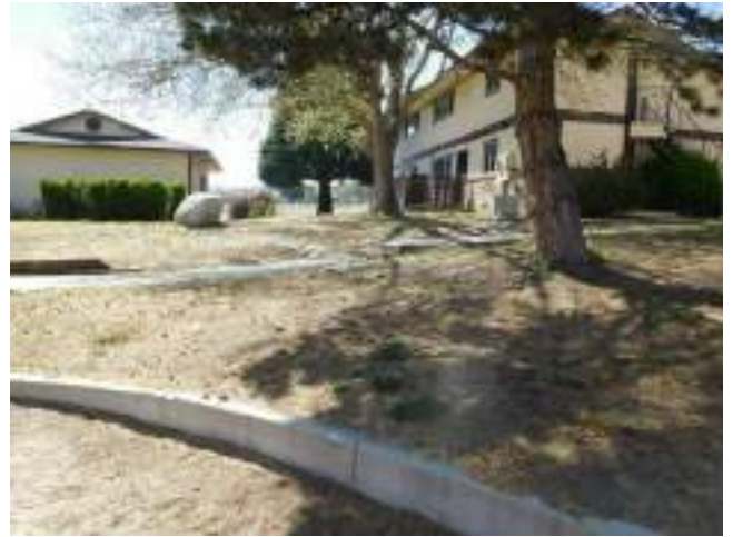
78. Area of bare ground at rear of maintenance garage (Non-Critical Repair)
