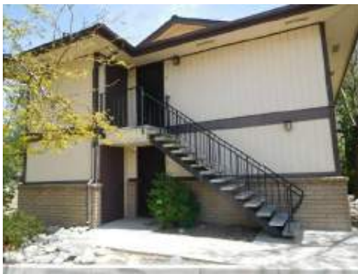
Upper floor unit access stairway at building end
