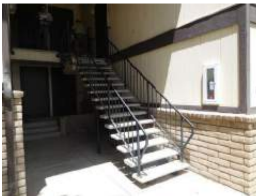
Upper floor unit access stairway at building connection
