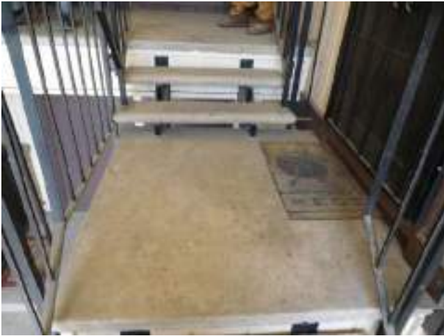
101. Typical stairway landing
