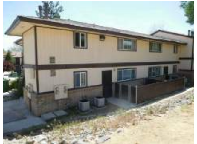
20. Typical exterior area
