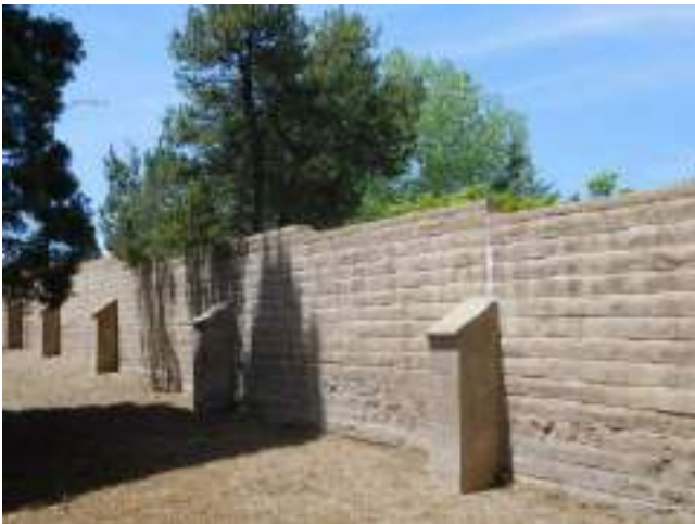
111. Partially retaining site wall at northern end of site
