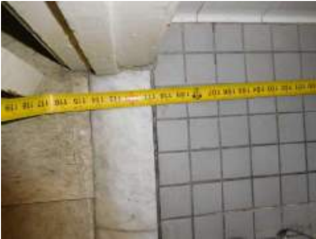
31. Bld 2541-Unit 1-2x1-UFAS -Bathroom
