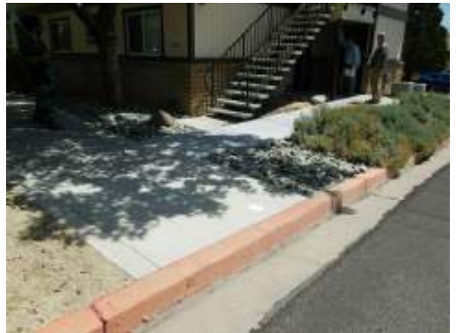
84. Typical flatwork termination at drive intersection
