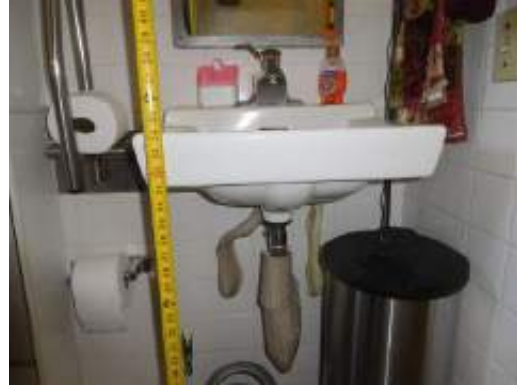
Bld 2541-Unit 1-2x1-UFAS -Bathroom
