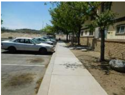
Typical flatwork in front of apartment building
