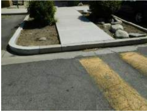
Typical flatwork termination at drive intersection
