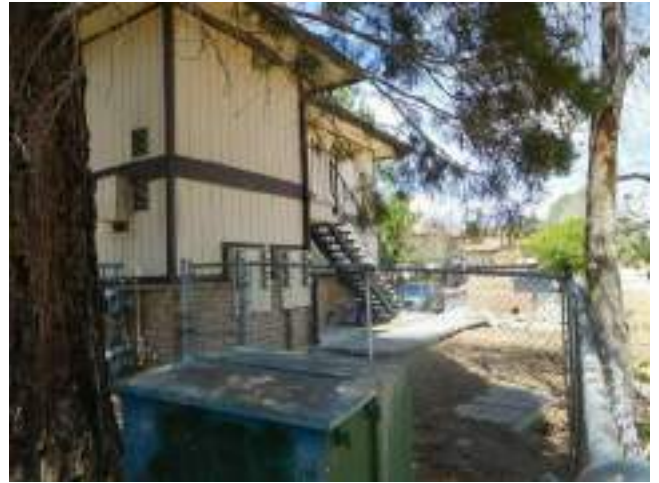
114. Chain link eastern perimeter fencing
