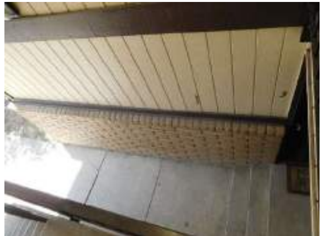
148. Connected building area stairwell cladding
