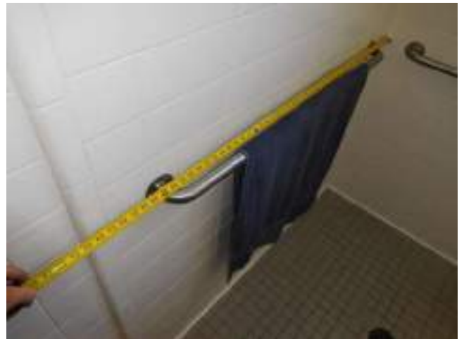
28. Bld 2541-Unit 1-2x1-UFAS -Bathroom
