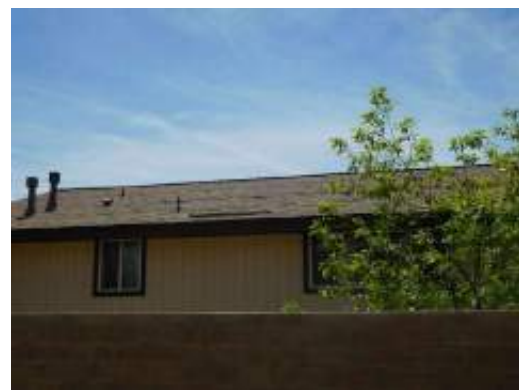
Typical roof condition
