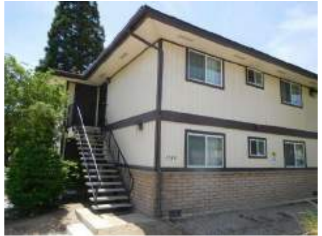
98. Upper floor unit access stairway at building end
