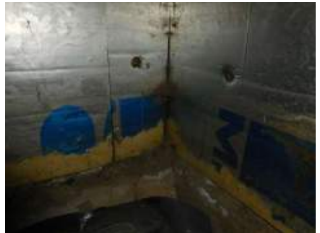
136. Representative crawl space with perimeter stem wall insulation
