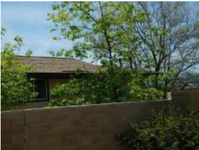
155. Typical roof condition
