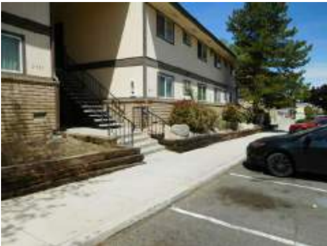
119. Landscaping timber retaining wall
