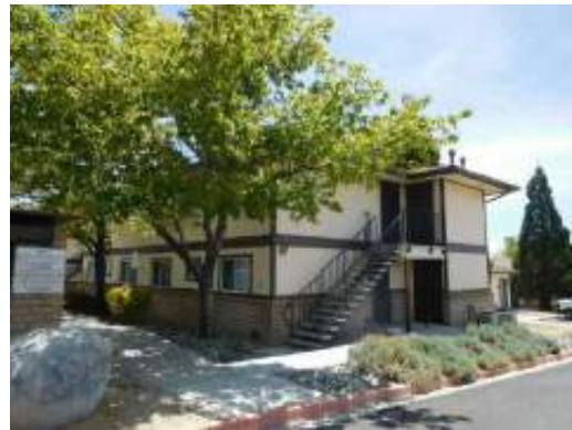
Typical exterior area
