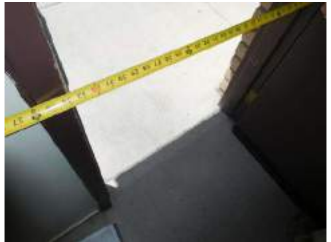
92. Laundry Room entrance
