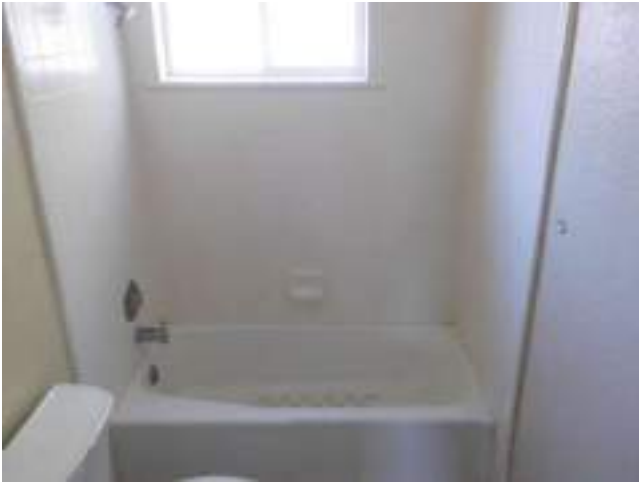
13. Bld 1512-Unit 3-2x1 -Bathroom
