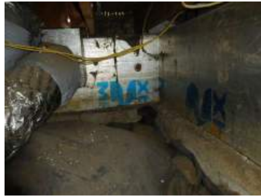
Representative crawl space
