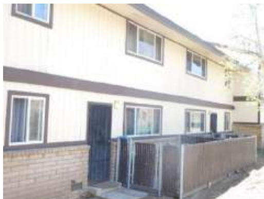
Unit rear doors
