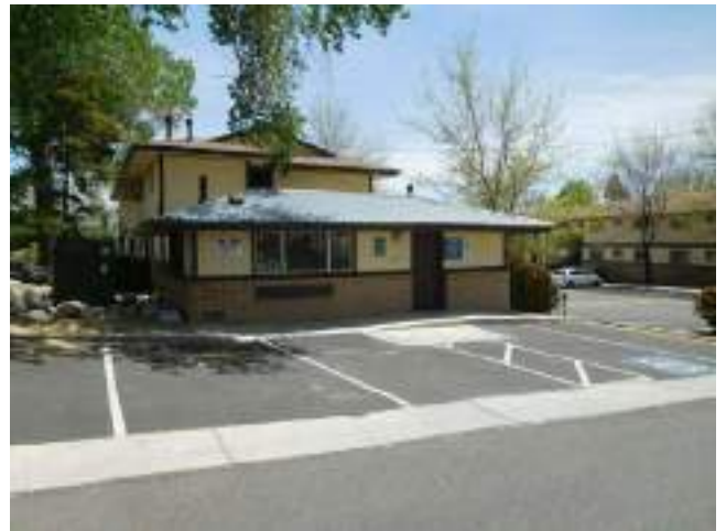
12. Typical exterior area at laundry building
