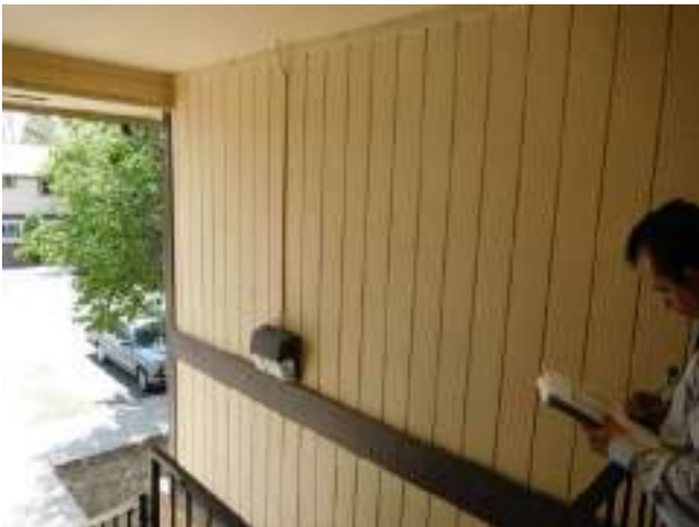
147. Connected building area stairwell cladding
