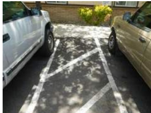
Typical ADA parking space at UFAS dwelling unit excessive slope and cross slope at access ramp (Critical Repair)
