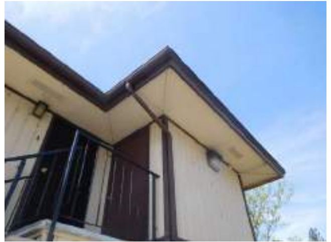
146. Facade with soffit venting
