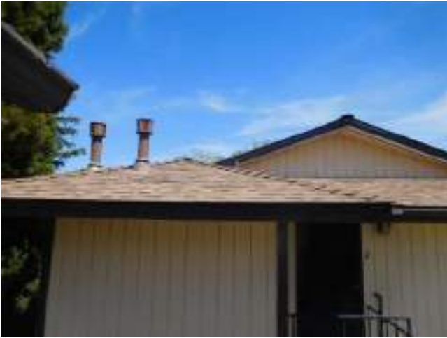
157. Typical roof condition
