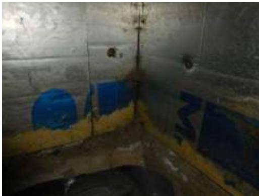
Representative crawl space with perimeter stem wall insulation
