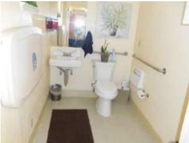
43. Leasing Office Community Room bathroom
