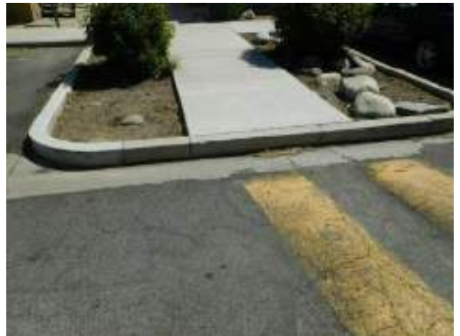
80. Typical flatwork termination at drive intersection
