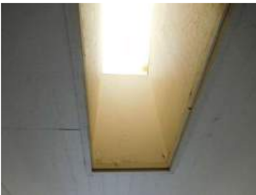
Typical roof skylight
