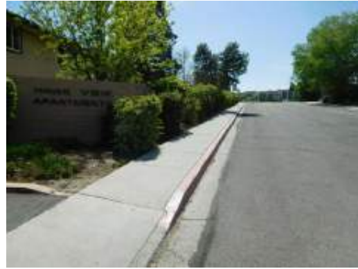
Flatwork site access northern end of site
