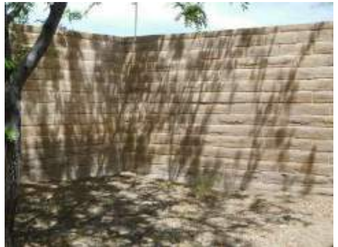
108. Partially retaining site wall at northern end of site
