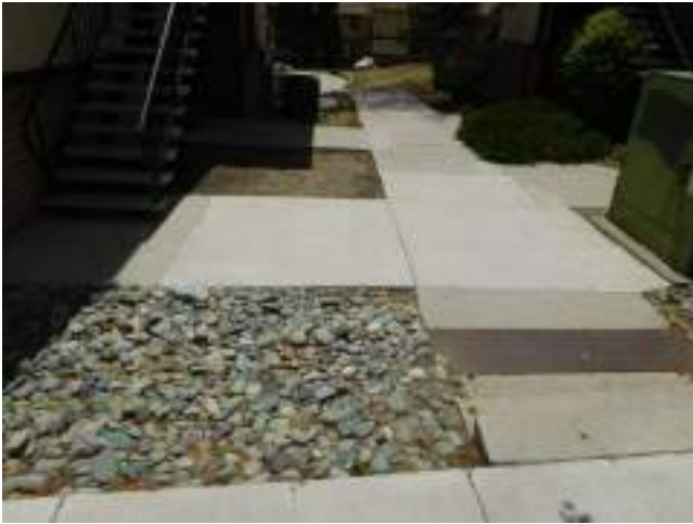
85. Area of flatwork sectional repair
