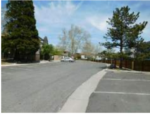
Typical asphalt paving
