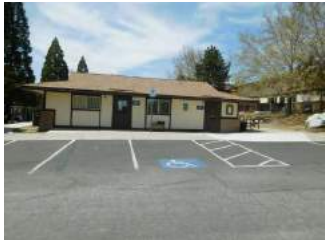
24. Leasing Office front with ADA parking space, non-van accessible (Critical Repair)
