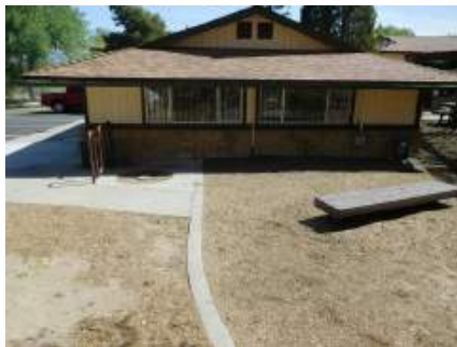
Leasing Office side
