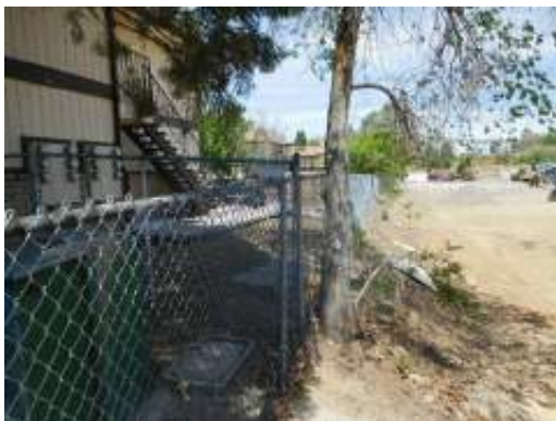
Eastern side of site at southern corner
