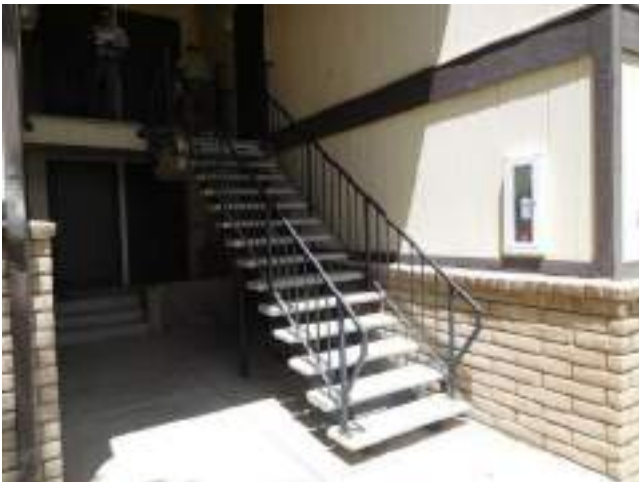
99. Upper floor unit access stairway at building connection
