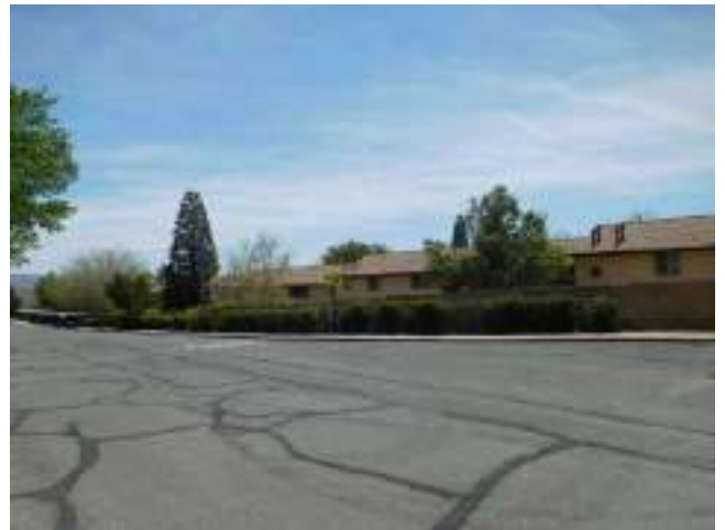
4. Northern end of site
