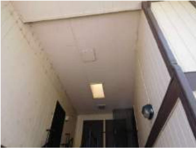
149. Connected building area stairwell cladding and roof skylight
