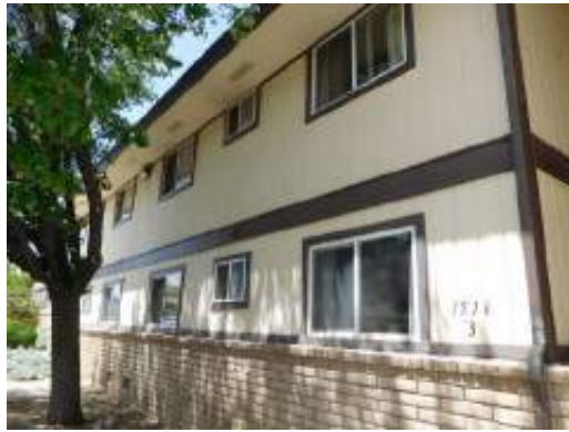
Typical window units
