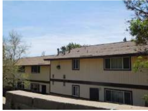
Typical roof condition
