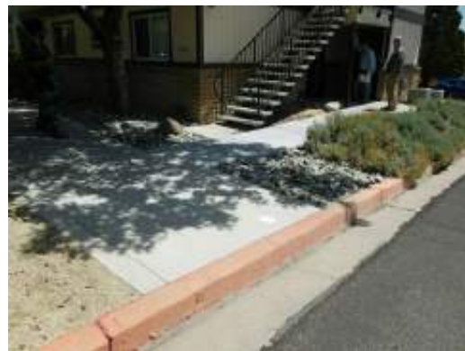
Typical flatwork termination at drive intersection
