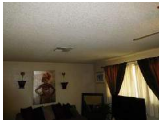
Typical drywall damage from building settling
