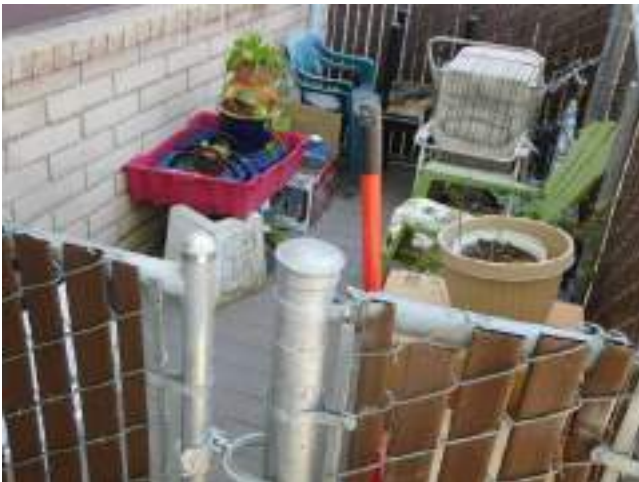
123. Ground level rear deck enclosed with chain linked fencing
