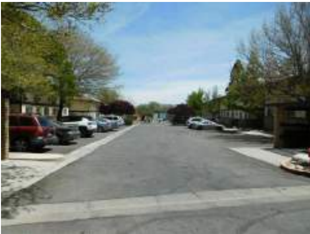
67. Typical asphalt paving
