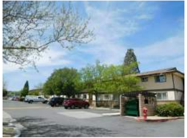
18. Typical exterior area
