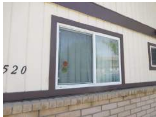
Typical window unit
