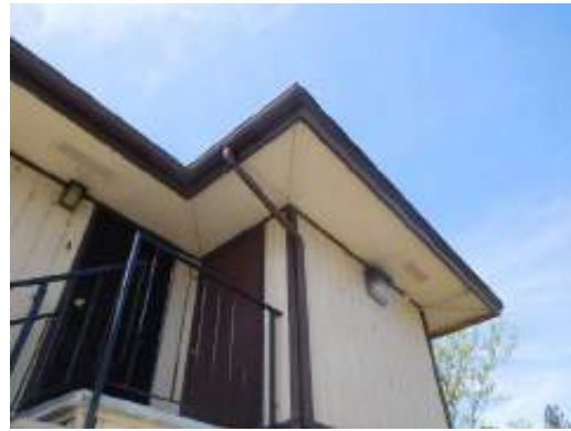
Facade with soffit venting
