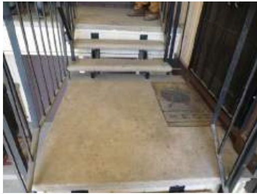
Typical stairway landing
