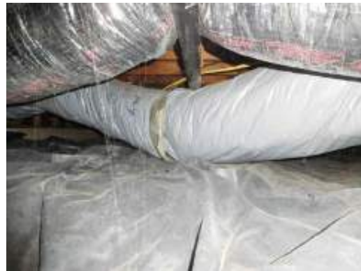
Representative crawl space with wood floor joists and moisture barrier
