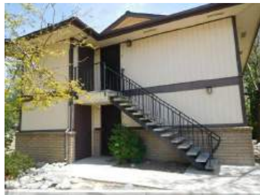
Upper floor unit access stairway at building end
