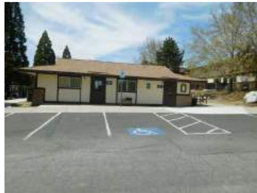
Leasing Office front with ADA parking space, non-van accessible (Critical Repair)
