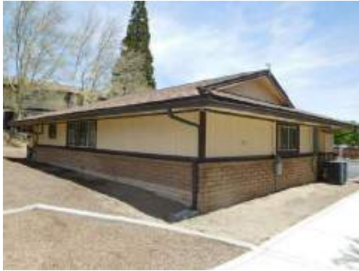
Leasing Office rear
