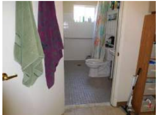
20. Bld 2541-Unit 1-2x1-UFAS -Bathroom
