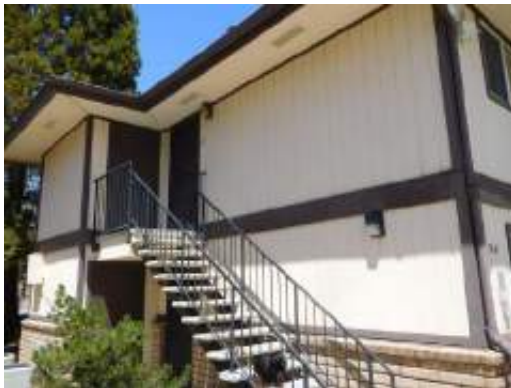
Apartment building end facade
