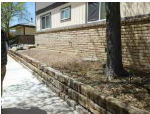
Landscaping timber retaining wall
