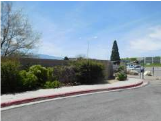
107. Partially retaining site wall at northern end of site
