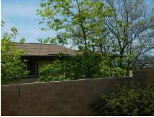
Typical roof condition
