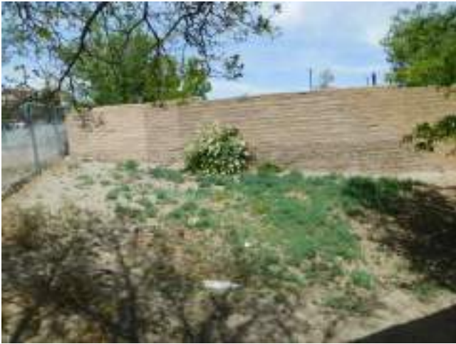
109. Partially retaining site wall at northern end of site
