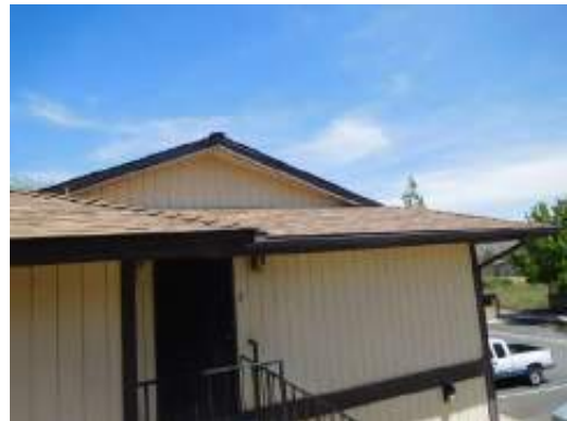
Typical roof condition
