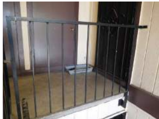
Dwelling unit and MEP room doors
