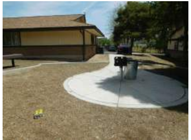
60. Rear of Leasing Office accessible access
