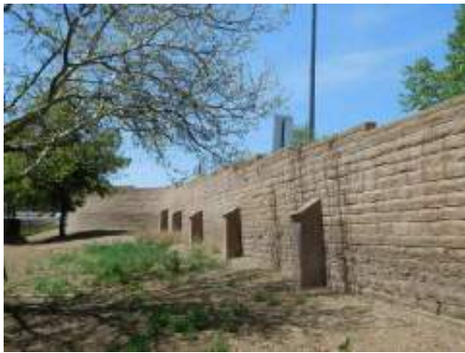
Partially retaining site wall at northern end of site
