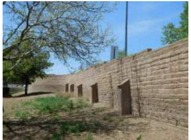
112. Partially retaining site wall at northern end of site
