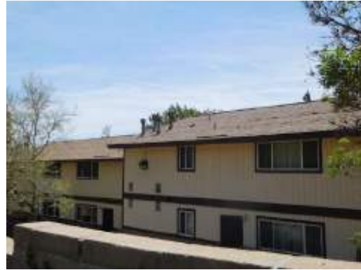
Typical roof condition
