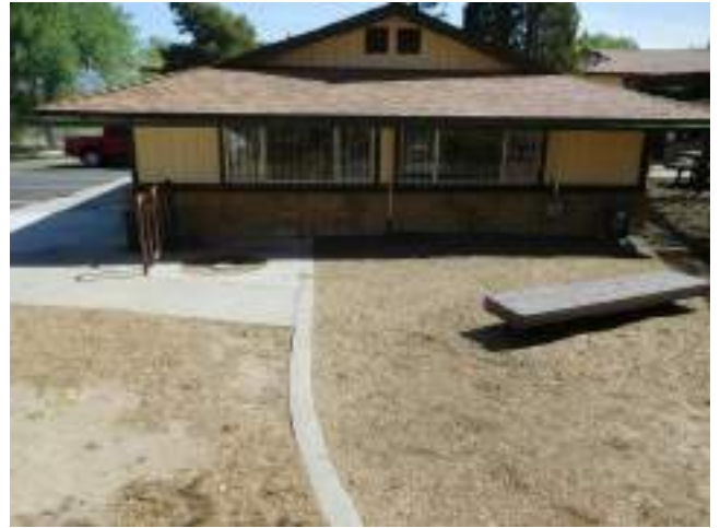
22. Leasing Office side
