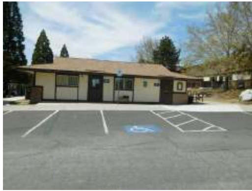
Leasing Office front with ADA parking space, non-van accessible (Critical Repair)
