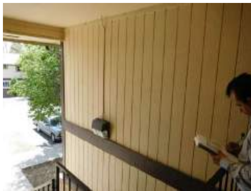
Connected building area stairwell cladding
