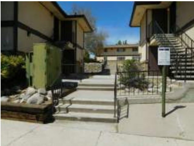
103. Site stairway between 2539 and 2545 Buildings
