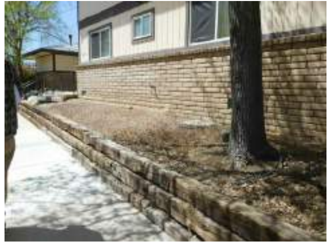
118. Landscaping timber retaining wall
