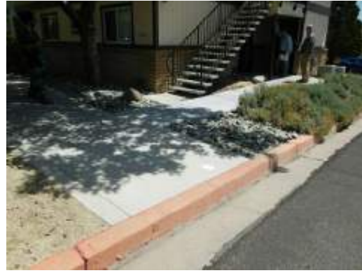
Typical flatwork termination at drive intersection
