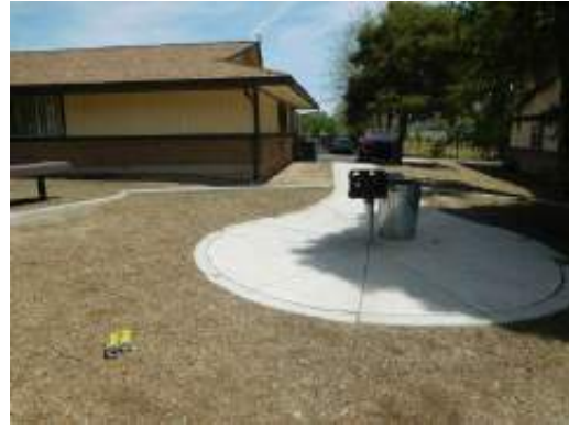
Rear of Leasing Office accessible access
