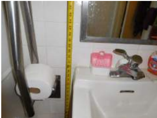
Bld 2541-Unit 1-2x1-UFAS -Bathroom
