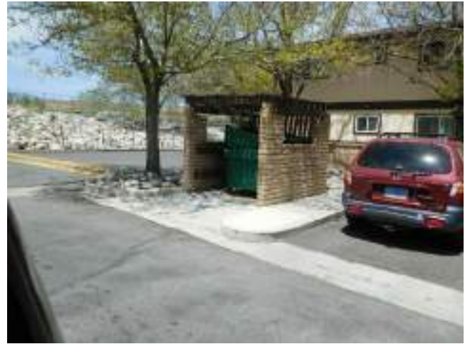
122. Refuse container with no accessible pathway (Critical Repair)
