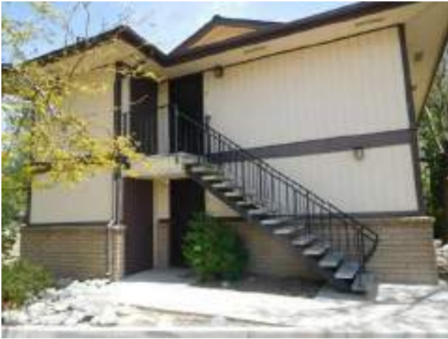
97. Upper floor unit access stairway at building end
