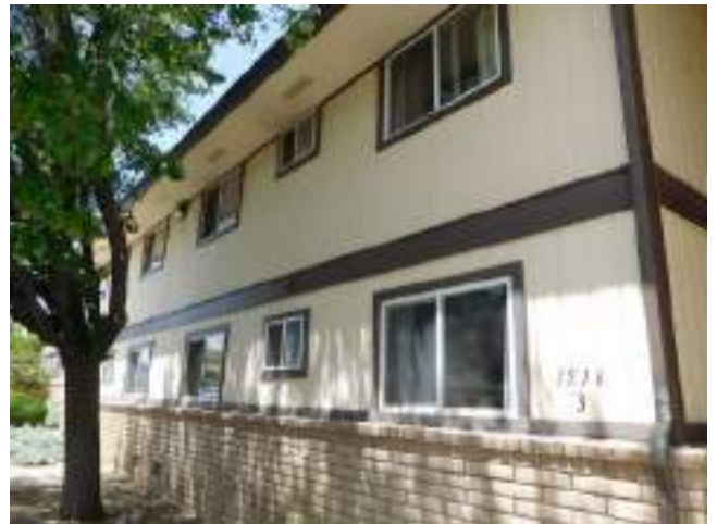
152. Typical window units
