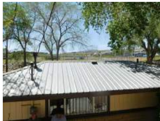
Laundry room metal panel roofing
