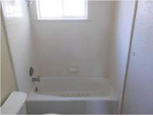
Bld 1512-Unit 3-2x1 -Bathroom
