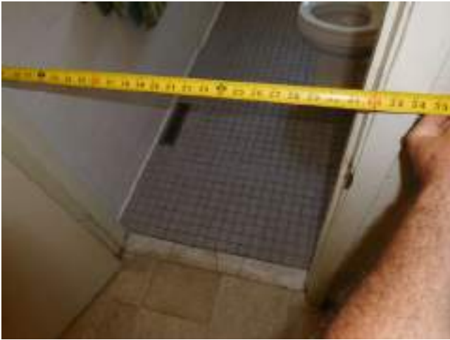
21. Bld 2541-Unit 1-2x1-UFAS -Bathroom
