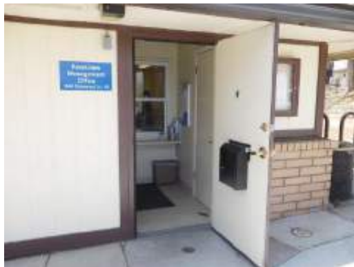
Leasing Office main entrance
