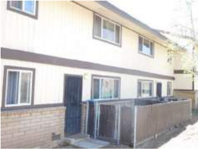
125. Ground level rear deck enclosed with chain linked fencing
