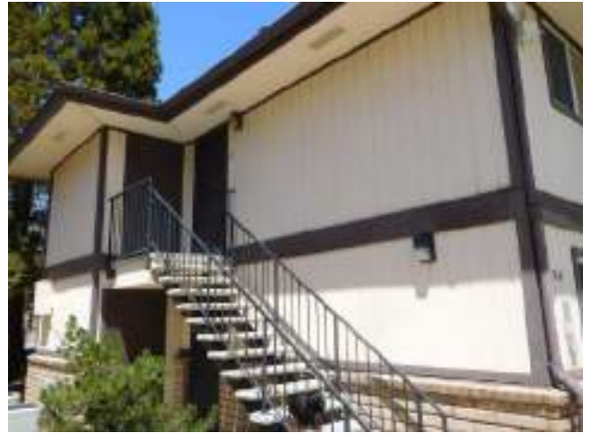
150. Apartment building end facade
