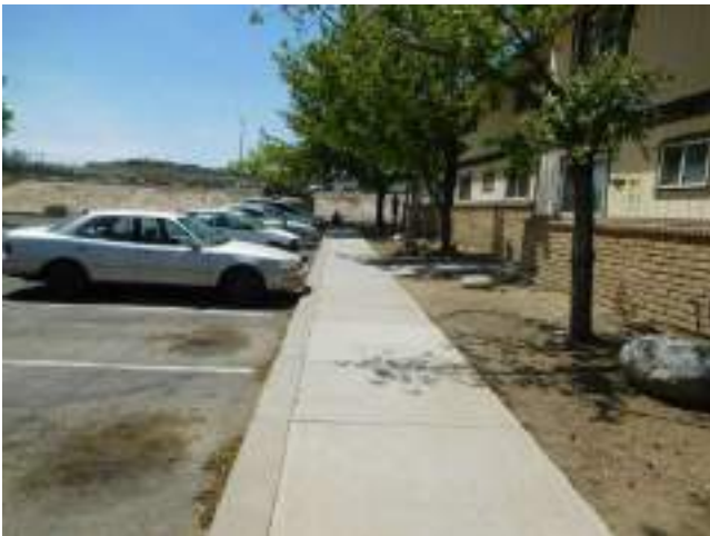
83. Typical flatwork in front of apartment building
