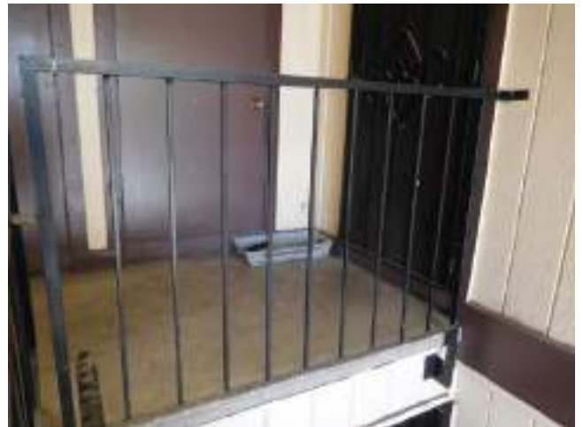
104. Typical onsite railing system
