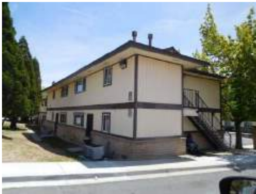
Typical exterior area
