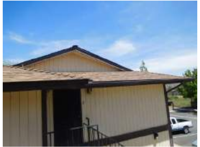
158. Typical roof condition
