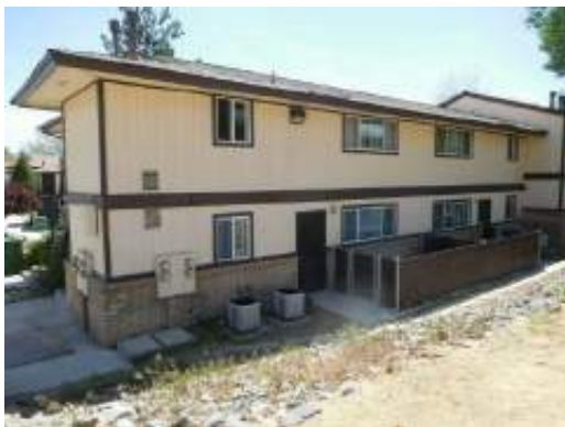
Typical exterior area
