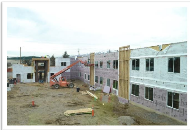
Construction on the Willie J. Wynn Apartments.
